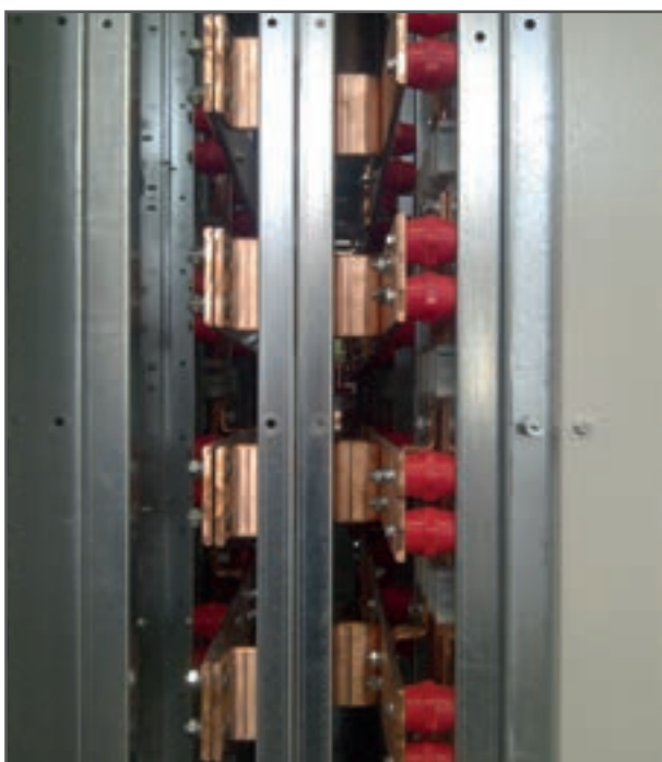
Colonna per adattamento quadri esistenti back to back Bck to back column for adaptation of existing switchboard Cellule pour adaptation des tableaux existents dos à dos
