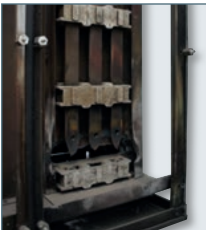
Vano sbarre / Bus bar compartment Compartment jeu de barres
