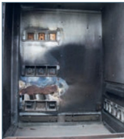
Cubicolo MCC / MCC cubicle MCC compartment
