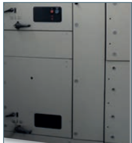
Quadro in prova / PMCC in test Tableau en preuve
